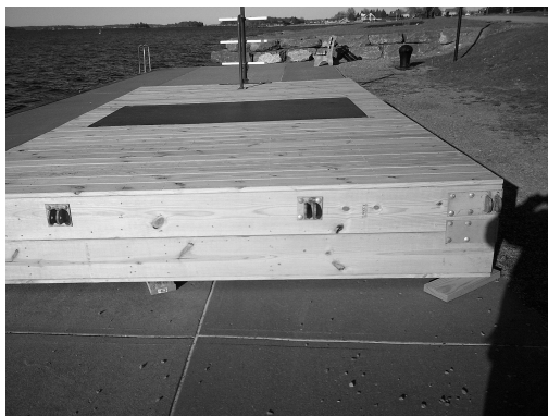
Diver's Access Platform Ready To Go Into The Water in Clayton
